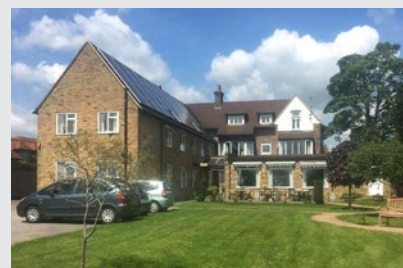
Alde House, Buckinghamshire
